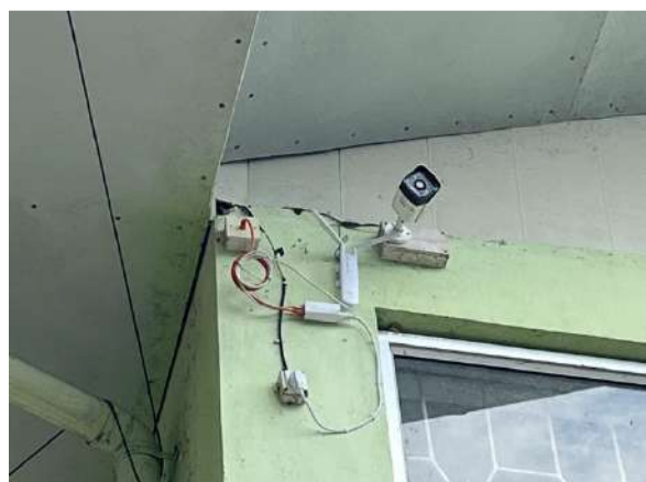
6. 01 no. of Outdoor Wi-Fi Router installed at Administrative Block, SGC, Rhenock.
