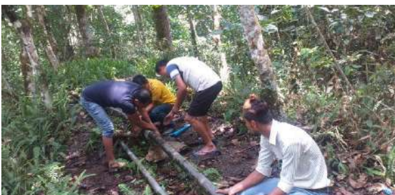
9. Main Line Pipe fitting at Rametey Dara at Chalisey.
