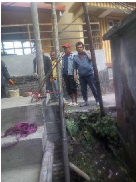
28. For support of 6 OFC Wire, Iron pole installed at Rungdung, Rhenock.
