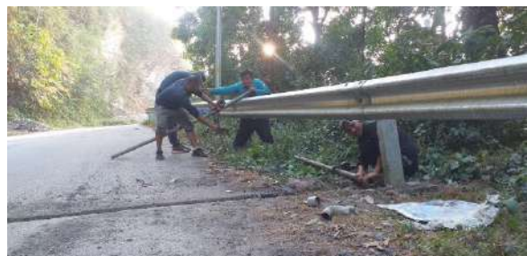
4. Main Line Pipe Road Crossing at Engineering Dara High Way near Chalisey.
