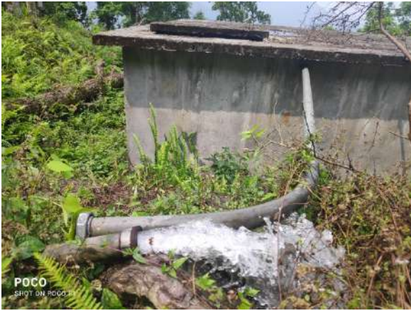
11. College Reserve Tank 2 Lakhs Litter Capacity.
