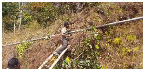
10. Main Line Pipe Fitting at Rametay Dara.
