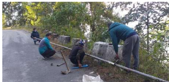
6. Main Line Pipe fitting at Engineering Dara near Chalisey Main Road.
