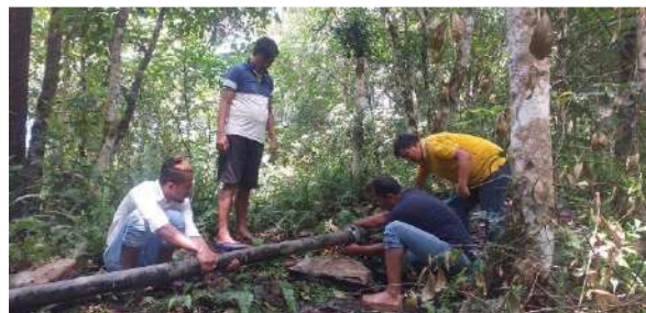
8. Main Line Pipe fitting at Chain Dara Chalisey
