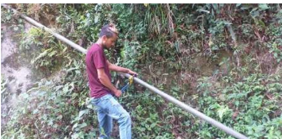
3. Main line pipe fitting above Engineering Dara.
