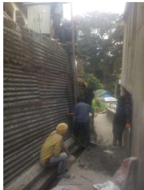
29. For support of 6 OFC Wire, Iron pole installed at Rungdung, Rhenock.
