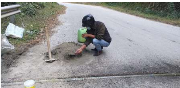
5. Filling of Digging portion at Engineering Dara.
