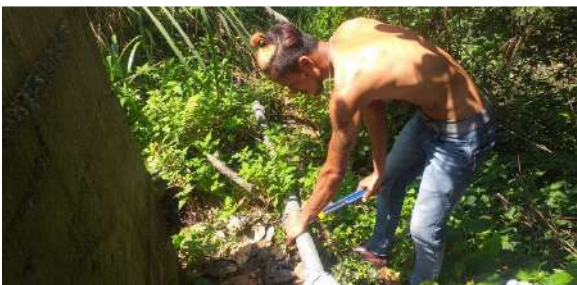
7. Mainline Pipe fitting at Engineering Dara.
