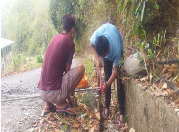
13. Road Crossing near D and B Block.
